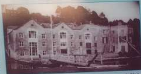
The Thames & Severn Headquarters after they had been converted to a polytechnic. We think this photo was taken around 1913. Picture courtesy of the Stanley Gardner Collection
